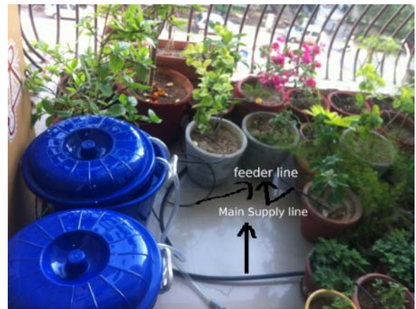
Fig. 6. Irrigation System Showing Installation of Pipes
