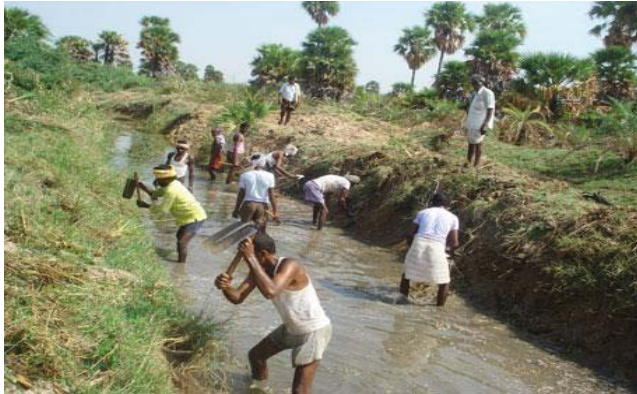
Figure 1 CHANNEL SYSTEM IRRIGATION
